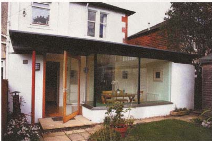
Above: The extension not only provides large, light, living areas but opens out on the garden; Left: The oak timber floors give a warm feel to the home, and cleverly designed window seats double as storage areas
